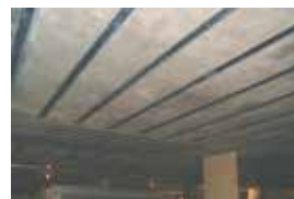
Example of floor slab strengthening
