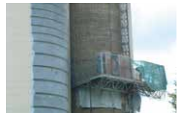
Example of silo strengthening
