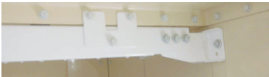
(Resin-coated reinforcement material used in the vapor phase area)
