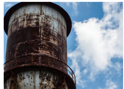
Metal corrosion
